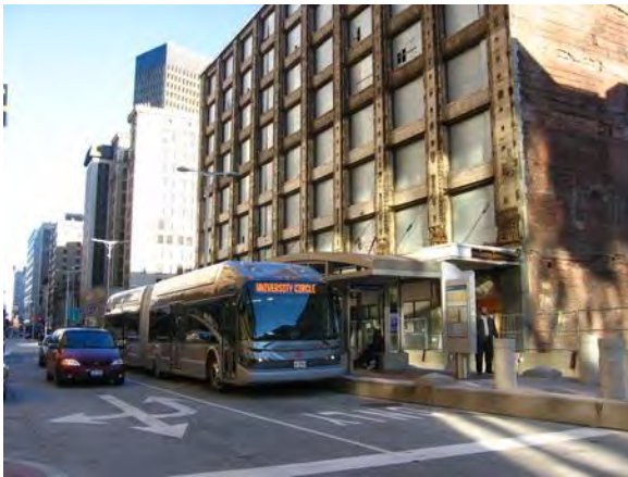
Renovation of 668 Building along HealthLine Route (source: Steven Litt)
