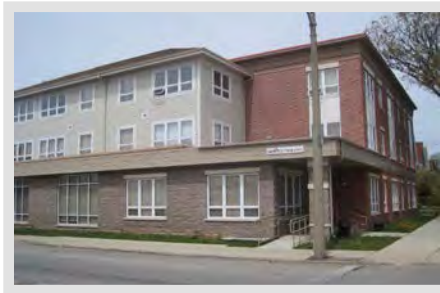
United House Christian Center, a 24-unit supportive housing development.
